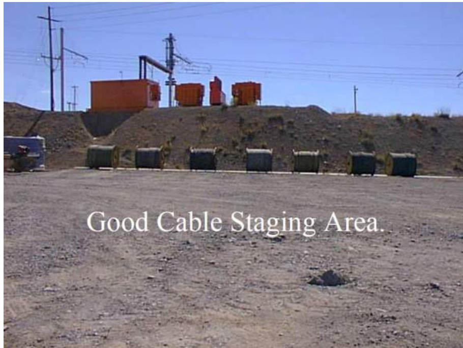
Figure 12: Cables are delivered to site ready to use.
